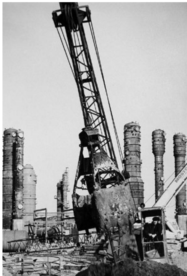
Rafineria Nafty Gdańsk w budowie / Oil Refinery in Gdańsk under construction
