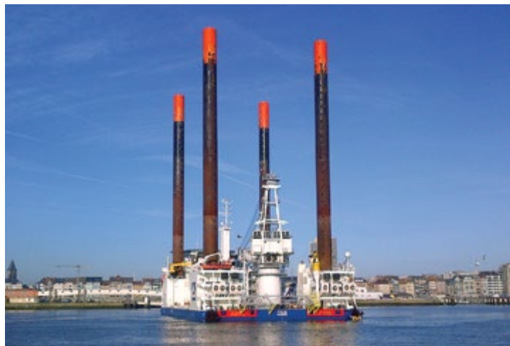
Platforma budowlano-remontowa Thor / Construction and repair platform Thor
