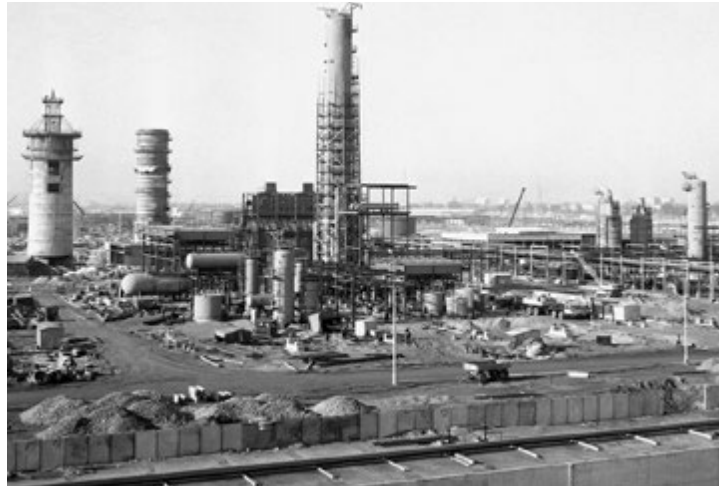
Rafineria Nafty Gdańsk w budowie / Oil Refinery in Gdańsk under construction
