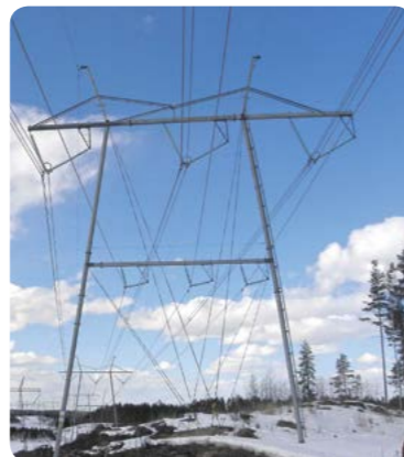
Linia dwutorowa 400 kV/110 kV Yllikkälä-Visulahti (Finlandia) / Double – circuit 400 kV/110 kV Yllikkälä-Visulahti (Finland) line
