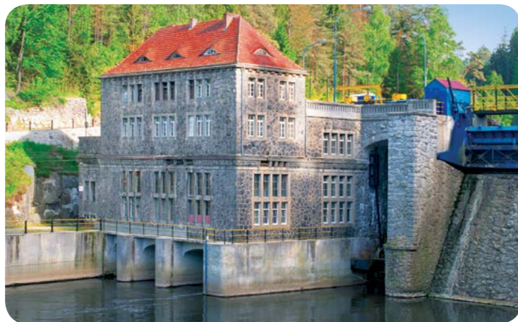
Elektrownia Wodna Bobrowice I z 1925 r. Bobrowice I Hydroelectric Power Plant built in 1925 (Tauron Ekoenergia)
