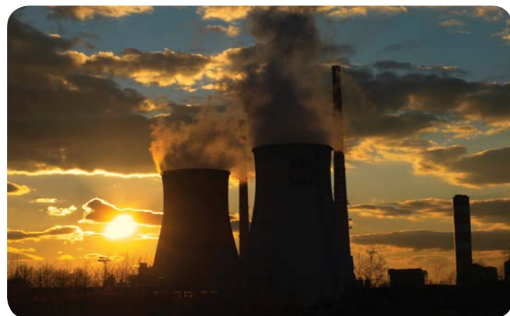
Elektrownia Rybnik – bloki energetyczne uruchomiono w latach 1972-1978 The Rybnik Power Plant – the power units were put into operation in 1972-1978 (arch. Photofactory®)
