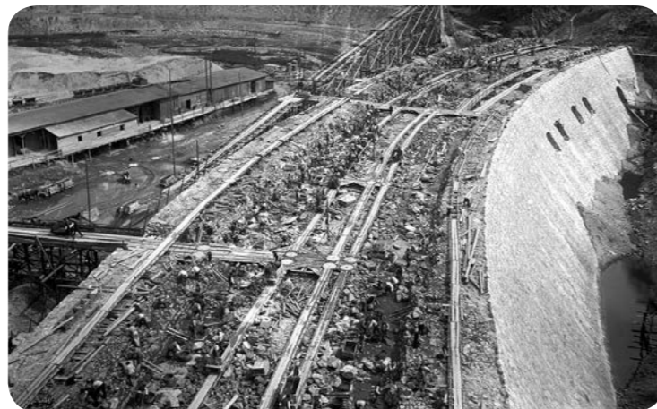
Budowa zapory w Pilchowicach – 1907–1912 r. / Construction of the dam in Pilchowice – 1907–1912 (arch. Photofactory®)
