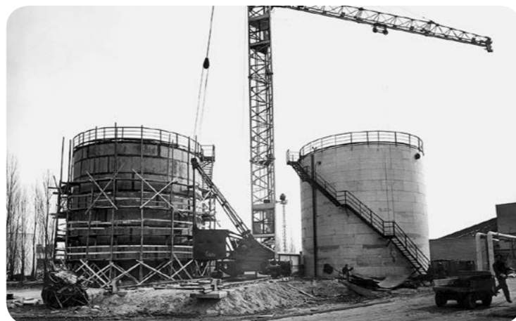
Budowa Elektrociepłowni Siekierki – 1959 r. / Construction of the Siekierki Thermal-Electric Power Station – 1959 (arch. Photofactory®)
