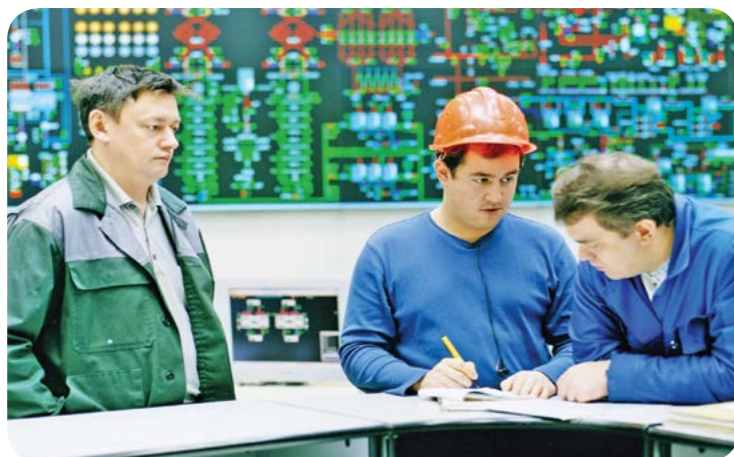
Elektrownia Jaworzno – nastawnia bloku / The Jaworzno Power Plant – power unit control room (arch. Photofactory®)
