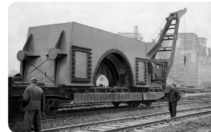
Budowa Elektrowni Turów – 1966 r. / The construction of the Turów Power Plant – 1966 (arch. Photofactory®)
