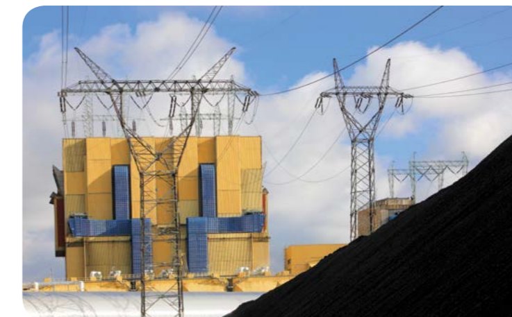
Elektrownia Kozienice – widok od strony nawęglania – kocioł bloku 560 MW The Kozienice Power Plant – a view from the carburizing plant – a boiler of the 560 MW unit (arch. Photofactory®)
