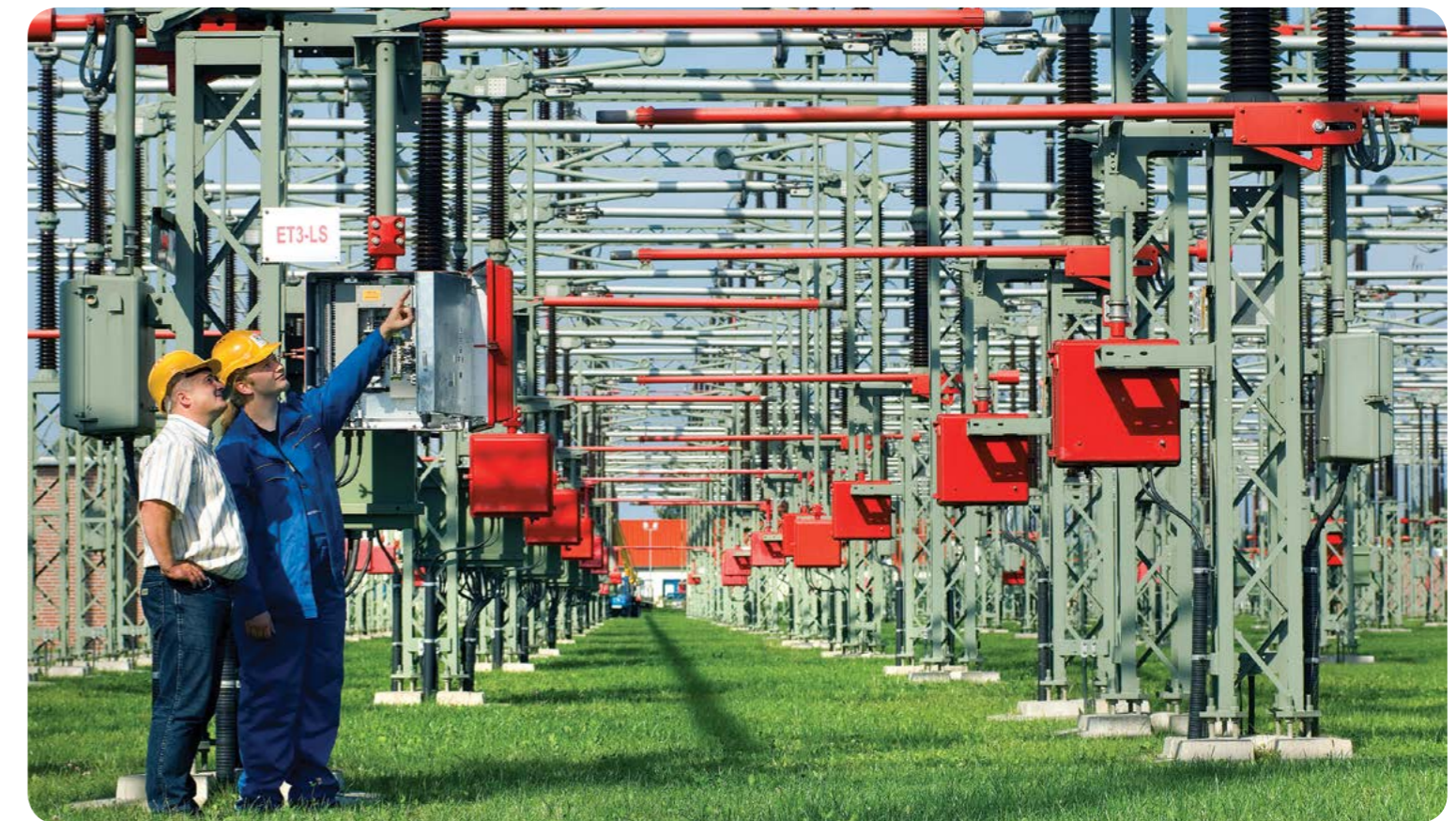
Zmodernizowana w 2010 r. SE Moszczenica 220/110/20/6 kV 220/110/20/6 kV Moszczenica switching station modernised in 2010 (arch. Photofactory®)
