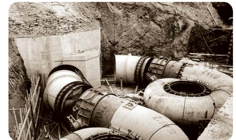
Transport elementów turbin do elektrowni wodnej (po lewej), fragment silnika opracowanego przez Jamesa Francisa (po prawej) Transportation of turbine elements to a hydroelectric power plant (on the left), a fragment of the engine designed by James Francis (on the right) (arch. Photofactory®)
