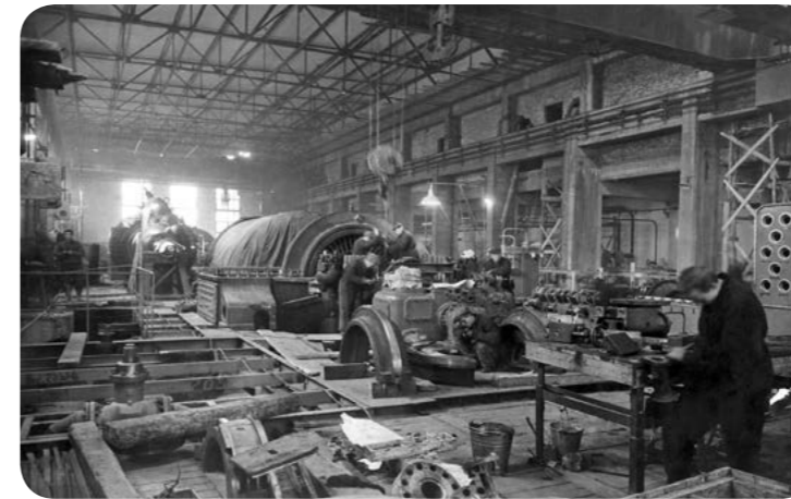
Elektrownia Jaworzno II – maszynownia, montaż turbiny – 1952 r. Jaworzno II Power Plant – engine house, installation of a turbine – 1952 (arch. Photofactory®)
