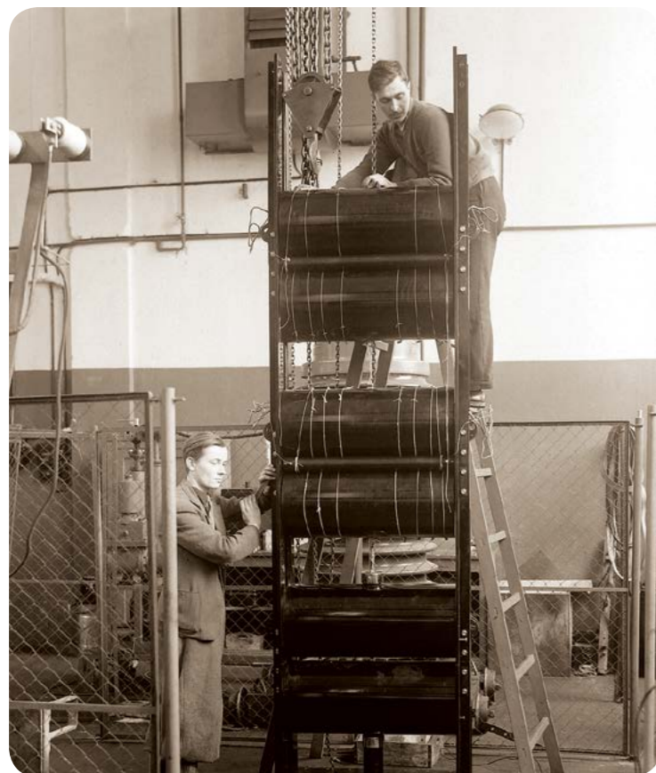
Kaskadowy transformator probierczy 450 kV / 450 kV cascade test transformer (arch. Photofactory®)
