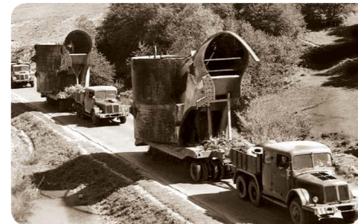
Transport elementów turbin do elektrowni wodnej (po lewej), fragment silnika opracowanego przez Jamesa Francisa (po prawej) Transportation of turbine elements to a hydroelectric power plant (on the left), a fragment of the engine designed by James Francis (on the right) (arch. Photofactory®)
