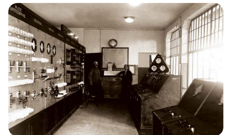
Nastawnia elektrowni Żur, 1936 r. / Control room of the Żur hydropower plant, 1936 (arch. Photofactory®)
