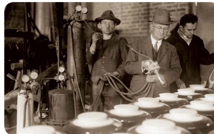
Metalizowanie izolatorów W60 / Metal plating of W60 insulators (arch. Photofactory®)
