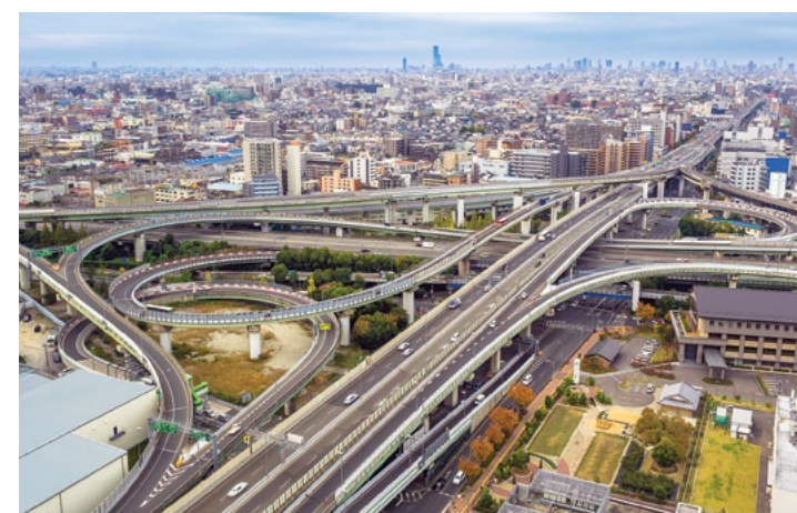
Autostrada Higashi Junction w Osace
