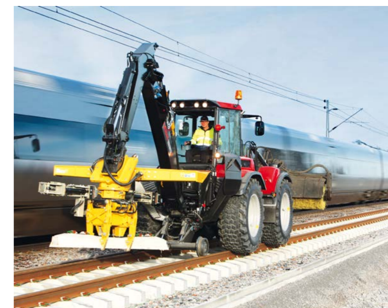
▲ Prace firmy BAMAAR | Works carried out by BAMAAR
